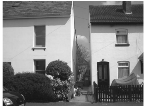
Figure 1: Grove Cottage (left) after refurbishment
