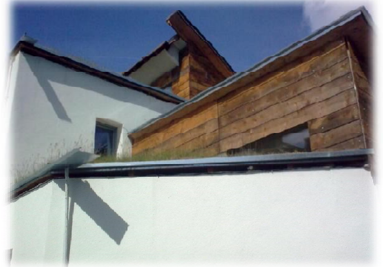
Grove Cottage: rear elevations (East)
